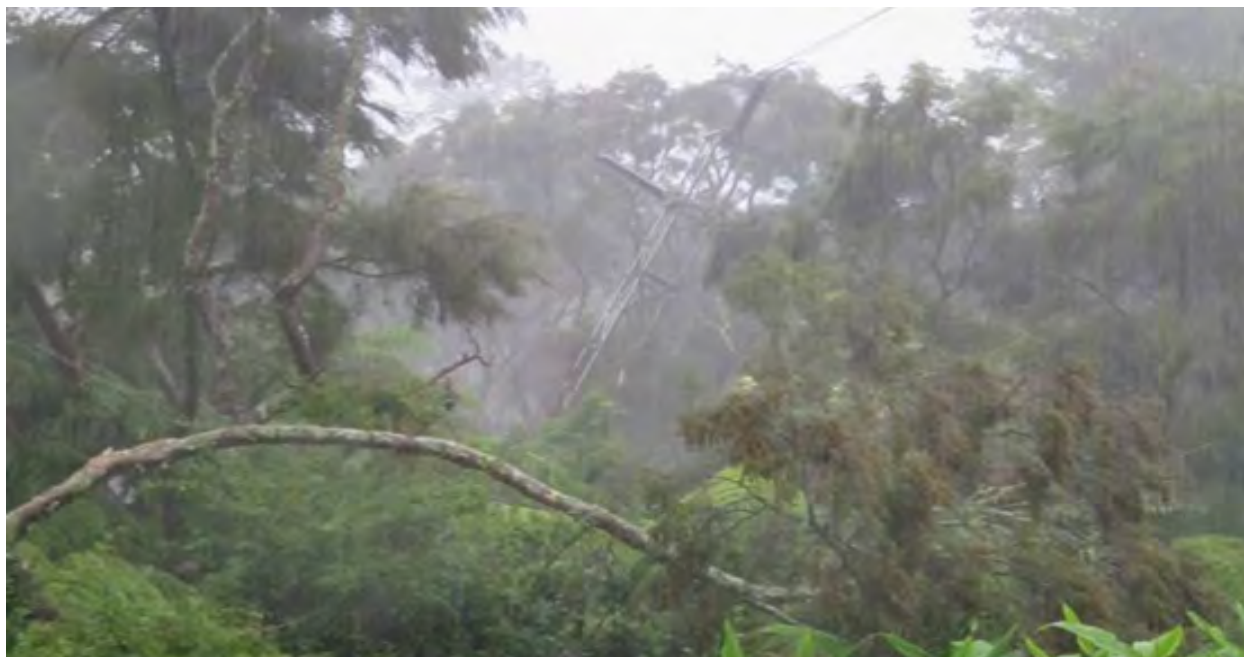
FIGURE 11.4: LEANING 110 KV SUBTRANSMISSION TOWER, GLENFIELD, JANUARY 2023
